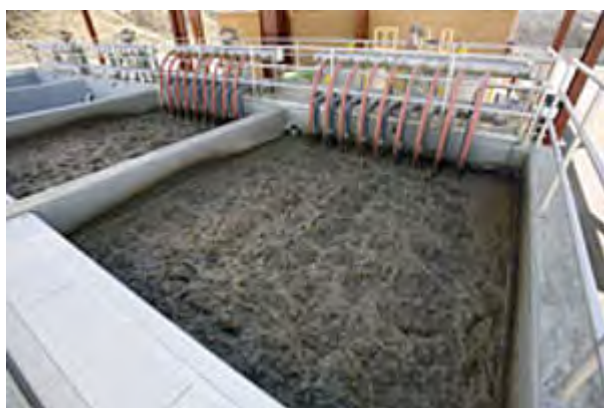
Fig. 2.4: Full-scale MBR plant with submerged membranes. Source: Spuhler 2011
