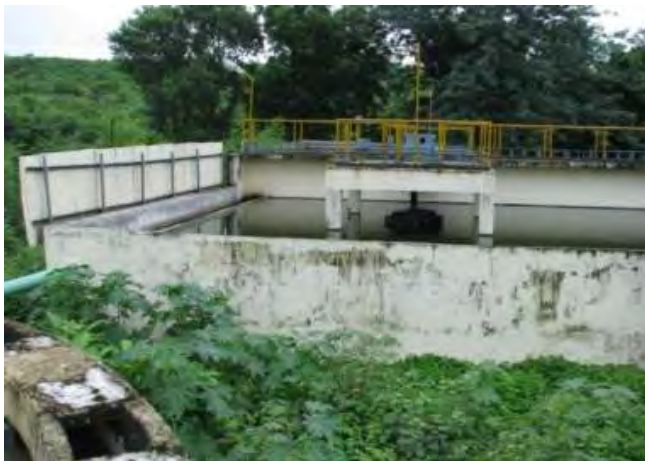
Fig. 2.1: Collapsed activated sludge wastewater treatment plant in Pandharpur, Maharashtra. Source: Barreto Dillon 2010
