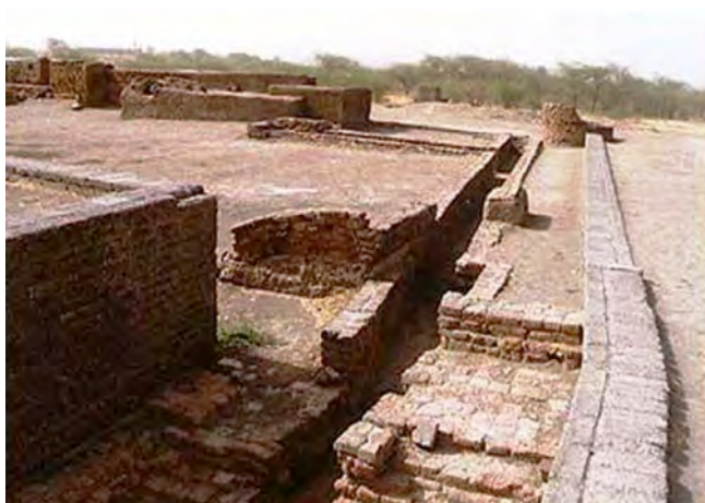
Fig. 1.2: Sanitary drain at Lothal, Indus Valley. The smoothened and joined brickwork made an intriguing yet efficient waste water treatment system discharging waste into the main sewer. Source: [Accessed: 10.07.2013]. http://www.sewerhistory.org/images/w/wam/loth_wam10.jpg
