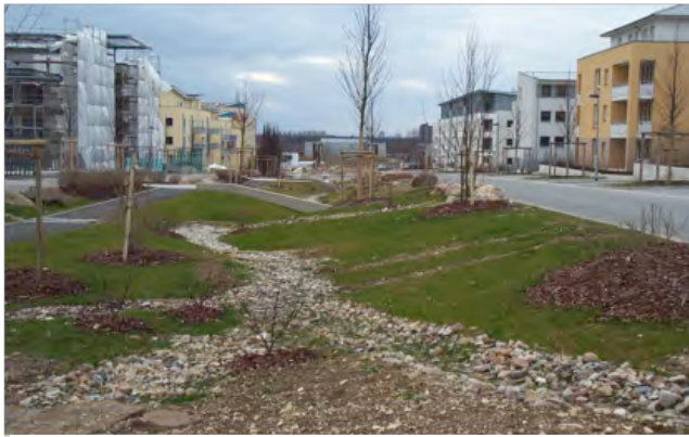
Fig. 2.2: Natural system for managed stormwater collection, treatment and infiltration in Switzerland. Source: Heeb 2008
