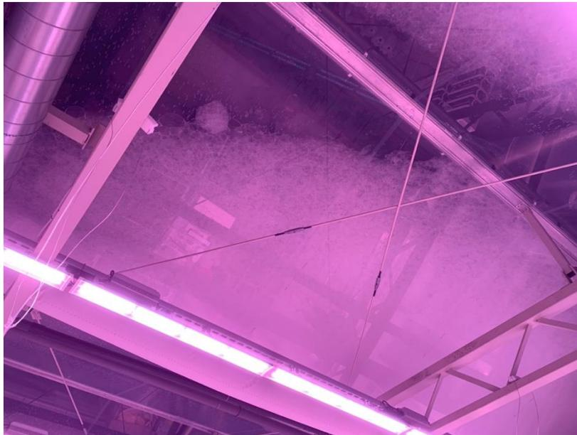
*Figure 4: Soap foam in the air space between two layers of plastic (roof)*
